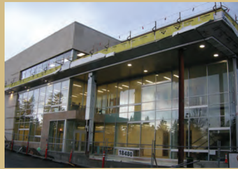
East County Courthouse
